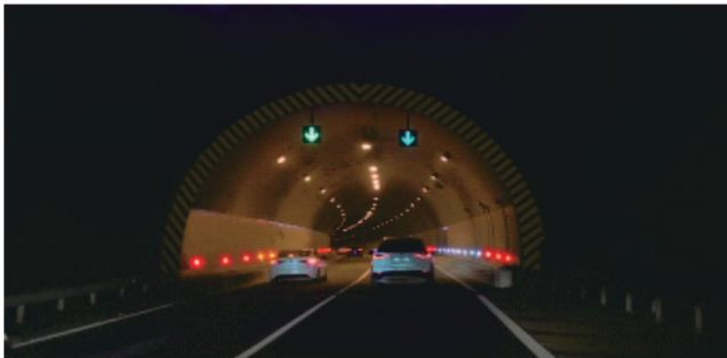
Assist in locating tunnel entrance vehicles
