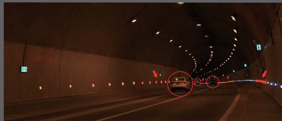
Assist in locating vehicles in tunnels
