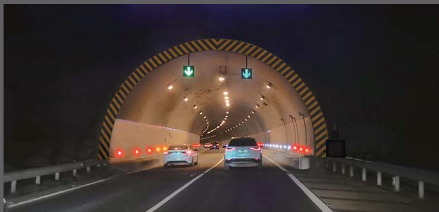
Assist in locating tunnel entrance vehicles
